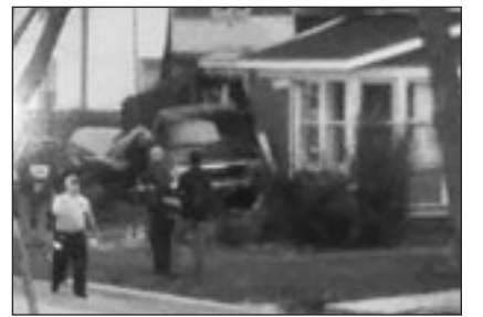
A truck backed into the front of this house in the 300 block of West Hawthorne Street in Elmwood last Saturday.
