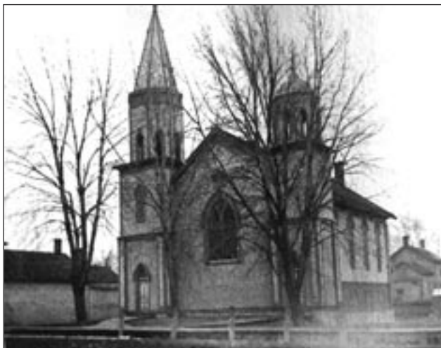
Pictured is the original Bradford First Baptist Church with the original bell tower, which was removed for safety reasons in 1908. Submitted photo.
