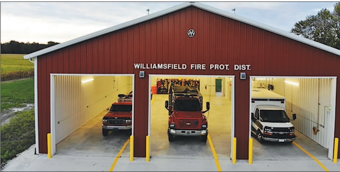
This addition is part of the remodeled Oak Run Fire Station that will be open to the public during an open house Saturday, July 10, from 10 a.m. to 2 p.m. Below is a new side-by-side that has been fitted with a new fire-medical skid courtesy of an Ameren Illinois grant. Submitted photos.
