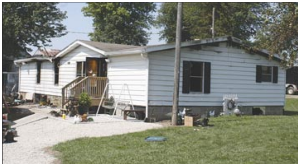
Shown is the Peterson house that still stands but was gutted by a fire early Monday morning, Aug. 30. Photo by John A. Ballentine.
