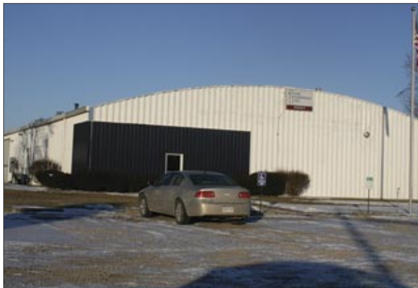
Pictured above is the former storage facility that will now house a new 10,000-square-foot fabrication shop for Bo/Gar Enterprises. Bo/Gar's second shop will include a new laser, welders and a brake press. Photo by John A. Ballentine.
