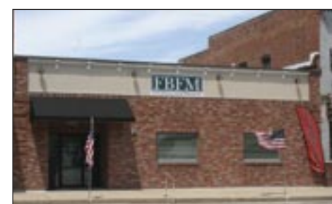
The FBFM building is located at 125 E. Main St. Photo by John A. Ballentine.
