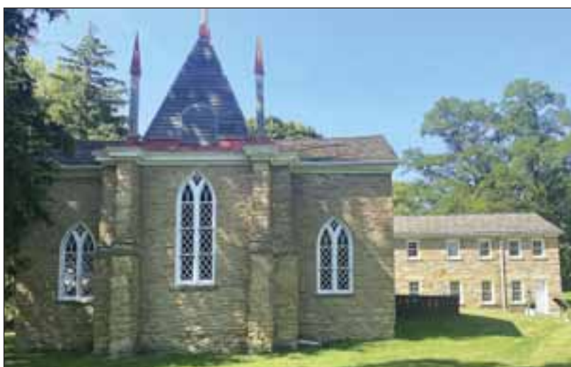
Made of hewn native stone, the south wing of Jubilee College (foreground) was built in 1839-40 and contains a chapel and classrooms. A west wing was added in 1842-44. Two other planned wings were never built. The site has recently reopened for tours Tuesdays through Saturdays from 9 a.m. to 5 p.m. Photo by Jeff Lampe.
