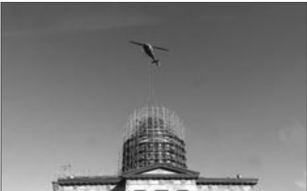
A helicopter is used to remove the flagpole from atop the Old State Capitol in Springfield on Monday morning as part of a renovation project to reinforce the dome and repair a leaky roof. Capitol News Illinois photo by Peter Hancock.
