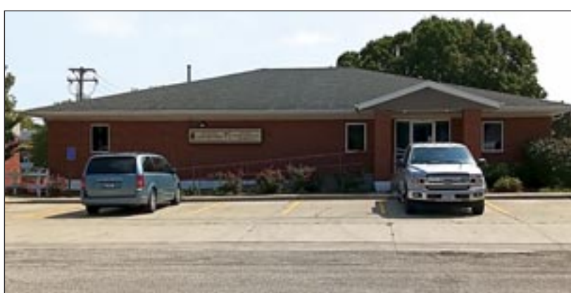
Pictured above is the planned location of Toulon’s new health care clinic, a joint effort of The State Bank of Toulon, First Choice Healthcare and Onero RX, Inc. expected to be completed in late fall. Photo by John A. Ballentine.
