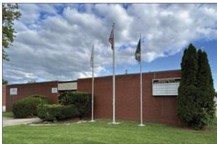
The Farmington City Council agreed to spend up to $400,000 for new HVAC systems at Farmington's Municipal Building at 322 E. Fort St. Photo by Jeff Lampe.
