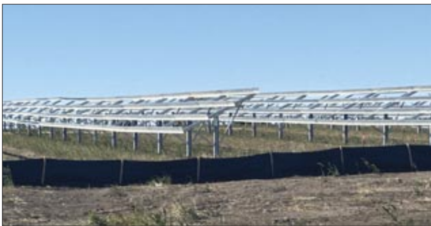
While this solar field south of Yates City has been completed, new projects are sprouting in fields across central Illinois. Photo by Jeff Lampe.
