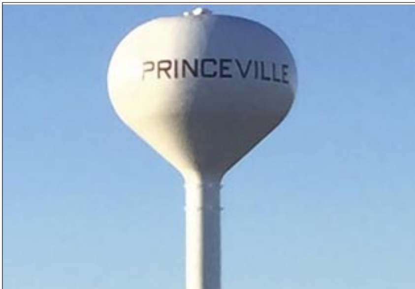
Officials in Edelstein and Princeville are hoping a federal grant will help pay for a 7-mile pipeline to bring Princeville water to Edelstein, whose current well is deficient.
