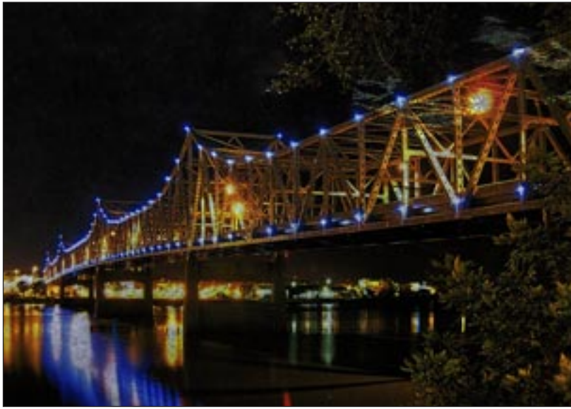
When the time came to replace lights on Peoria's Murray Baker Bridge as part of Upgrade 74 from 2002-06, H&H Industries, Inc., was part of the solution. Working with a California manufacturer and Oberlander Electric, H&H helped design 8-watt LED lights that saved energy and transformed the Peoria skyline by changing the color of the lights from orange to white.
