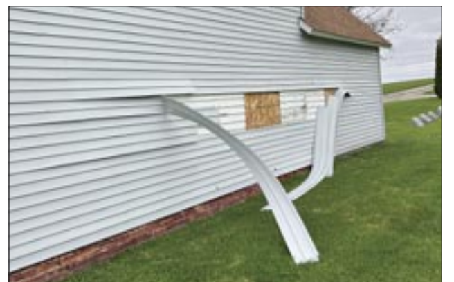
Siding on a building in Galva was damaged by an EF-1 tornado that passed through the city on Sunday. Photo by Carol Townsend.
