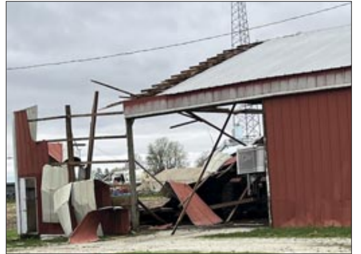
A farm building in Galva owned by Pete VanDeVelde suffered heavy damage from an EF-1 tornado that passed through the city Sunday evening. Photo by Carol Townsend.
