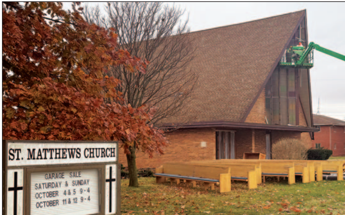
Workers from M&O Environmental Company of Peoria remove windows from the old St. Matthews Church in Farmington on Tuesday. Demolition of the church is expected to start soon.
