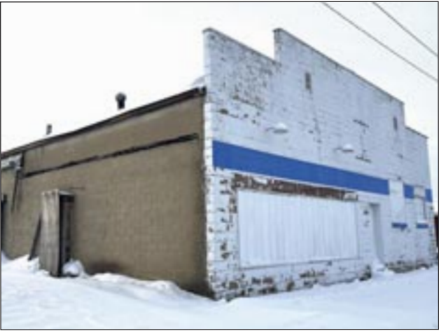
The former Lord Chevrolet building on Market Street in Galva has been a topic of conversation for the Galva City Council. Photo by Carol Townsend.
