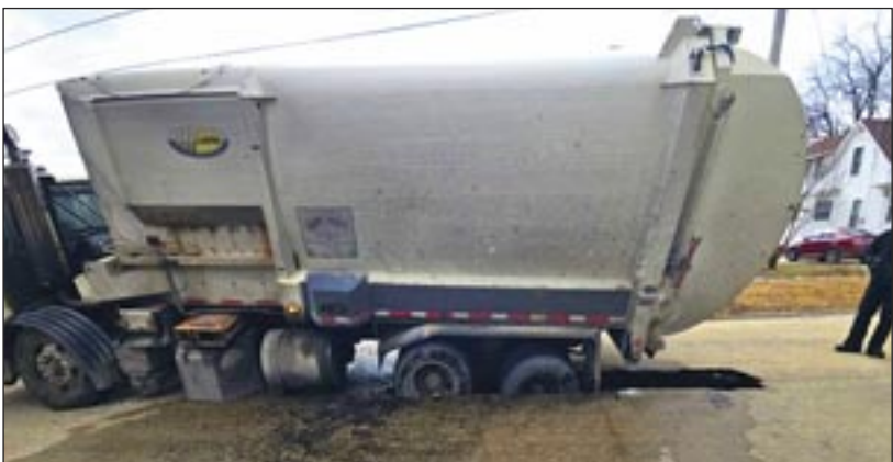
An Eagle Enterprises garbage truck fell through the pavement in the 400 block of NE 2nd St. in Galva last Wednesday. The pavement gave way after a sewer service line collapsed beneath the street.
